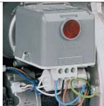
Control box fitted with an ignition transformer
